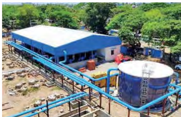
Figure 9.7: The Nesapakkam Plant to treat 10 MLD of wastewater
