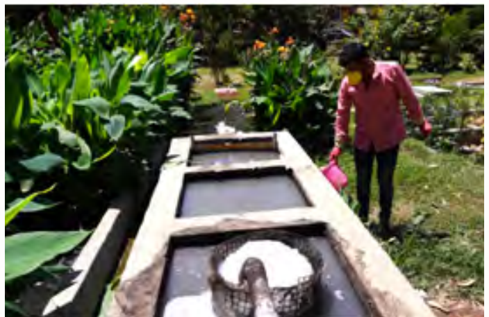
Figure 4.8: Phytorid technology type of wastewater system
