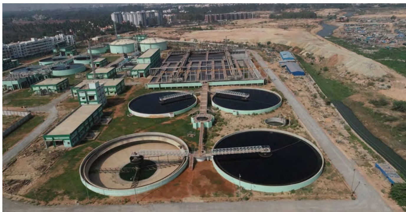
Figure 4.2: BWSSB Sewage Treatment Plant in Bellandur
