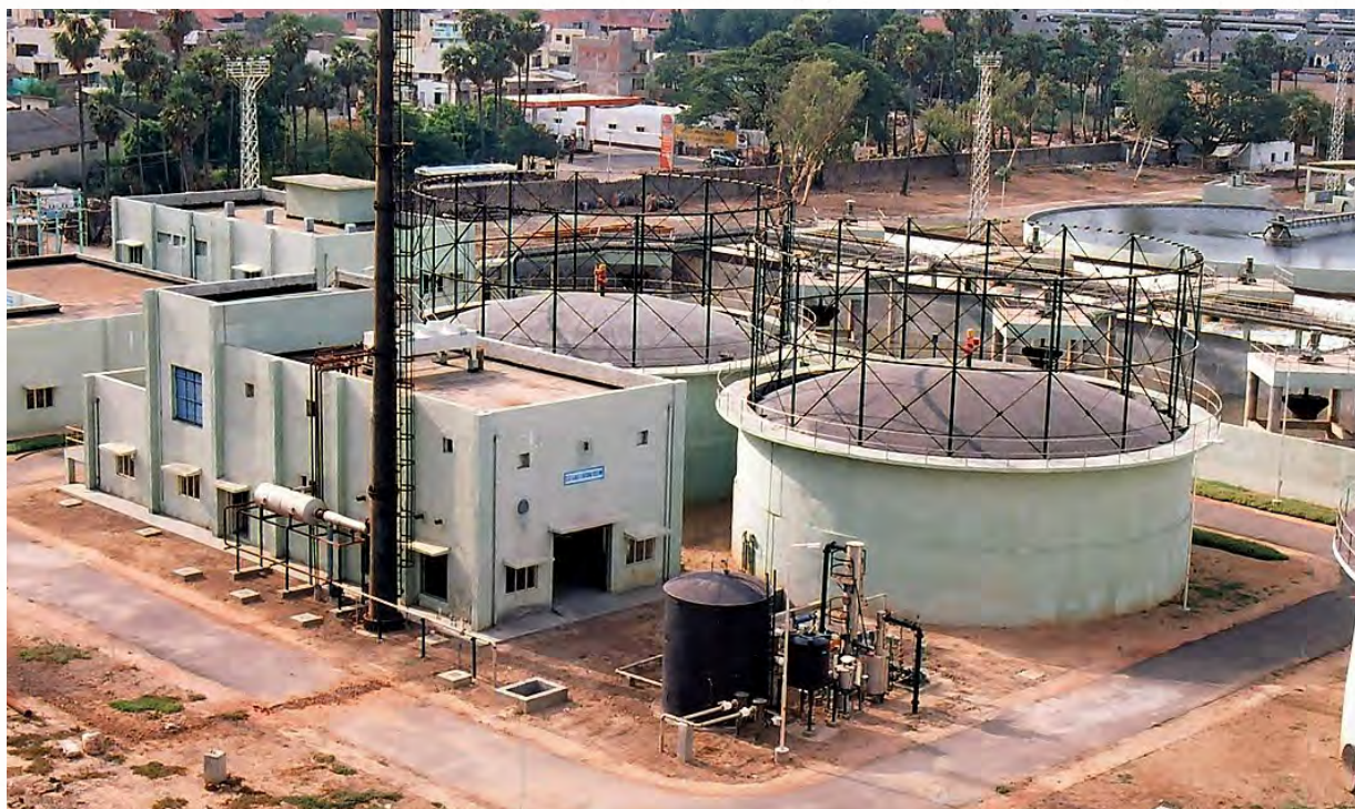
Figure 9.5: Koyambedu Sewage Treatment Plant
