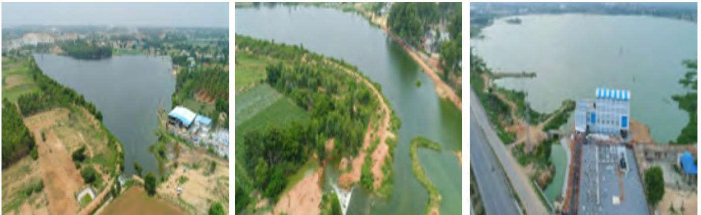
Figure 4.3: Uddapanahalli, Jodikrishnapura and Narsapura lakes filled with treated wastewater from KC valley project
